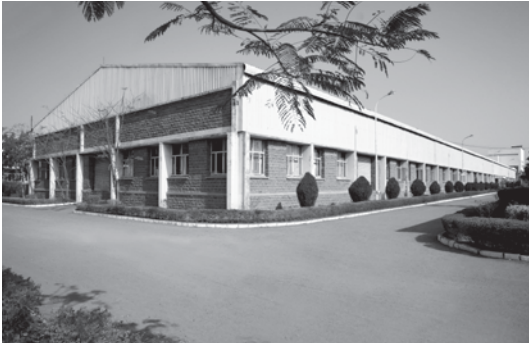
Wipro Furniture Manufacturing Facility at Waluj, Aurangabad, M.S. India.
